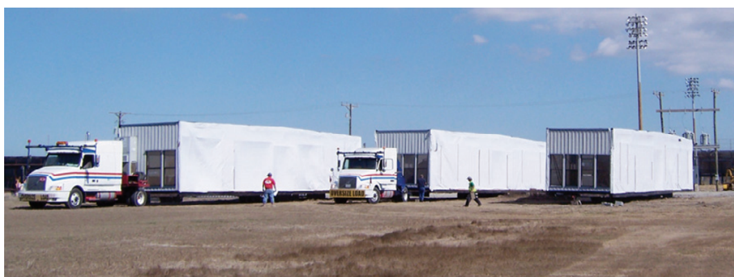
NEW TEMPORARY units for South Cameron High School have begun to arrive in Creole. Even the trucks were red, white and blue. The school was destroyed by Hurricane Ike. A temporary school facility is being operated in Lake Charles. (Photo by Cyndi Sellers.)
